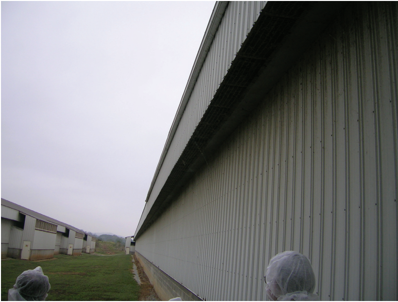
Fig. 7. Open eave along entire length of the poultry house to allow air entry to attic space prior to distribution to building interior.
